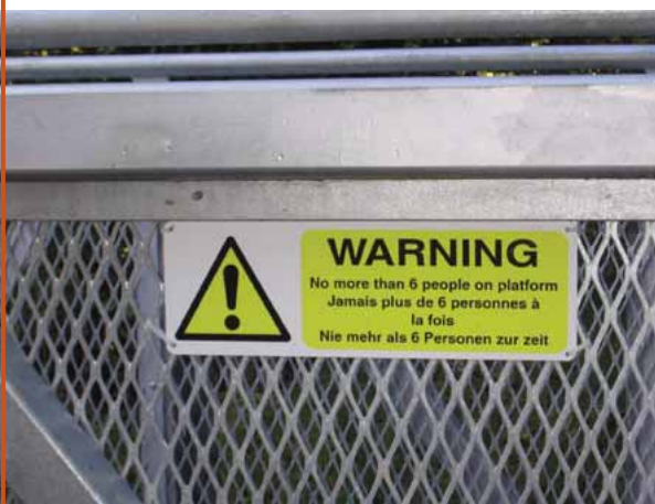
Bridge viewing platform with hazard sign
